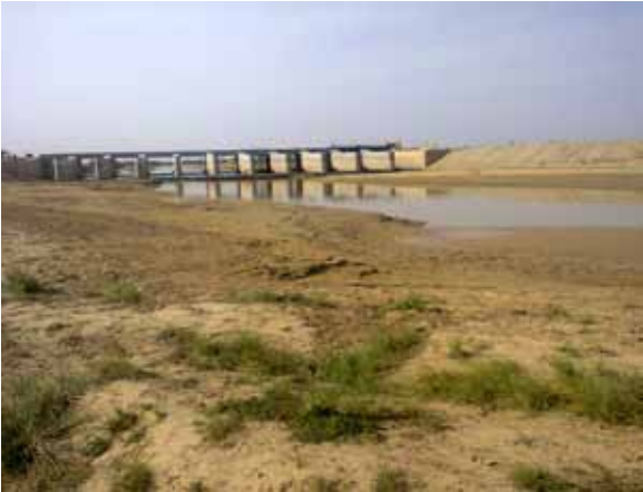
14.1 Haji Shahar mini barrage under construction Nari River Balochistan
