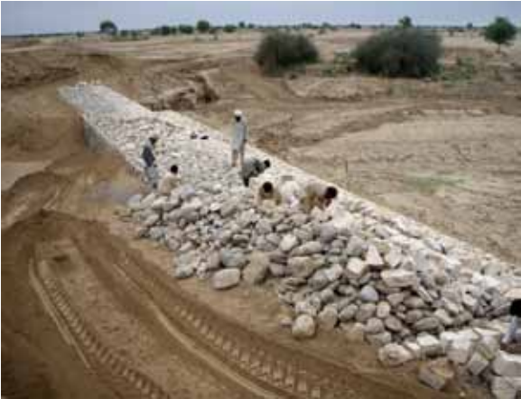
11.1 Construction of permeable spillway in earthen diversion bund
