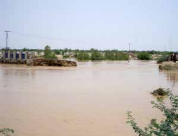
14.2 Damage after 2010 massive floods
