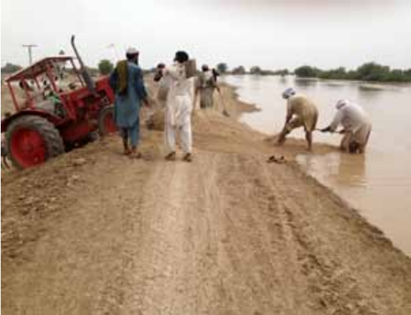
10.1 Plugging seepage hole in guide bund
