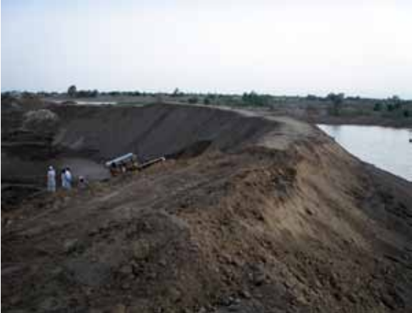
2.2 Repair of diversion bund D.I. Khan
